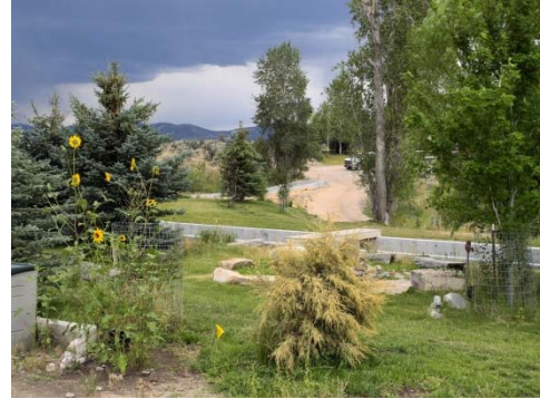
Example of Concrete Lined Channel (Near View)
