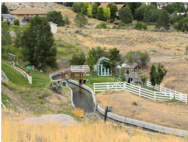
Existing Concrete Canal through Residential Development
