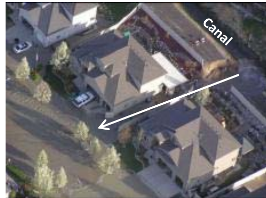
Canal Breach in Murray, UT (Image courtesy of KSL news)
