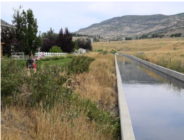
Existing Concrete Canal Adjacent to Residential Development
