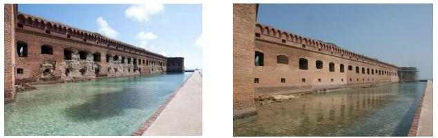
Before and After: Front 3 Comprehensive stabilization of upper and lower embrasures; removal of existing iron Totten shutter assemblies; infill arch reconstruction, replicated shutter component installation; scarp repointing as well as parapet brick replacement and repointing.
