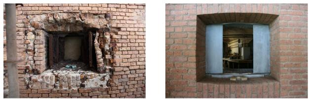
Before and After: Front 3 Lower Level Bastion Embrasure Reconstruction including removal of existing corroded iron Totten shutter assembly components and installation of replicated shutter components along with brick replacement and repointing.
