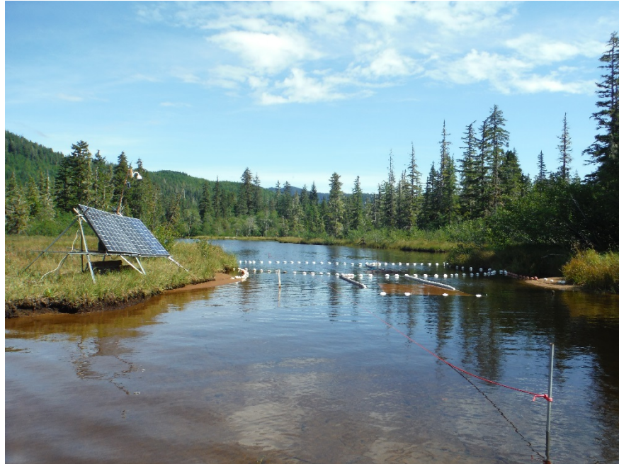
Figure 3. Pair of remotely monitored swim-through video net weirs at the outlet of Sitkoh Lake, 2016.
