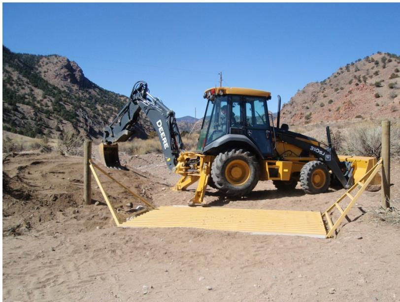
Installation of a cattleguard, in cooperation with the Colorado Parks and Wildlife, is used to provide access to the Arkansas Headwaters Recreation Area and prevent livestock from getting out onto the highway.
