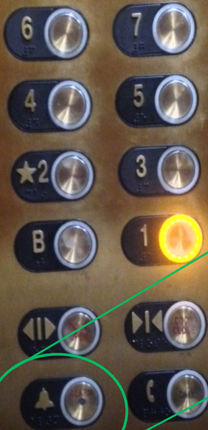
Left Side Control Panel
