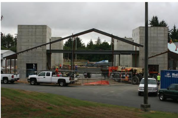
Construction of the first engineered tsunami refuge takes place in Westport, WA, in 2015. The completed tsunami refuge will span the flat roof of a gymnasium (9 meters above ground), with doors at ground level providing access to stairs within the corner towers. Photo credit: Sonya Miller, Ocosta School District
