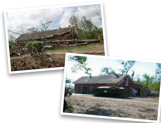
Historic carriage house damaged by Hurricane Katrina before and after stabilization, Chalmette, LA. (NPS)
