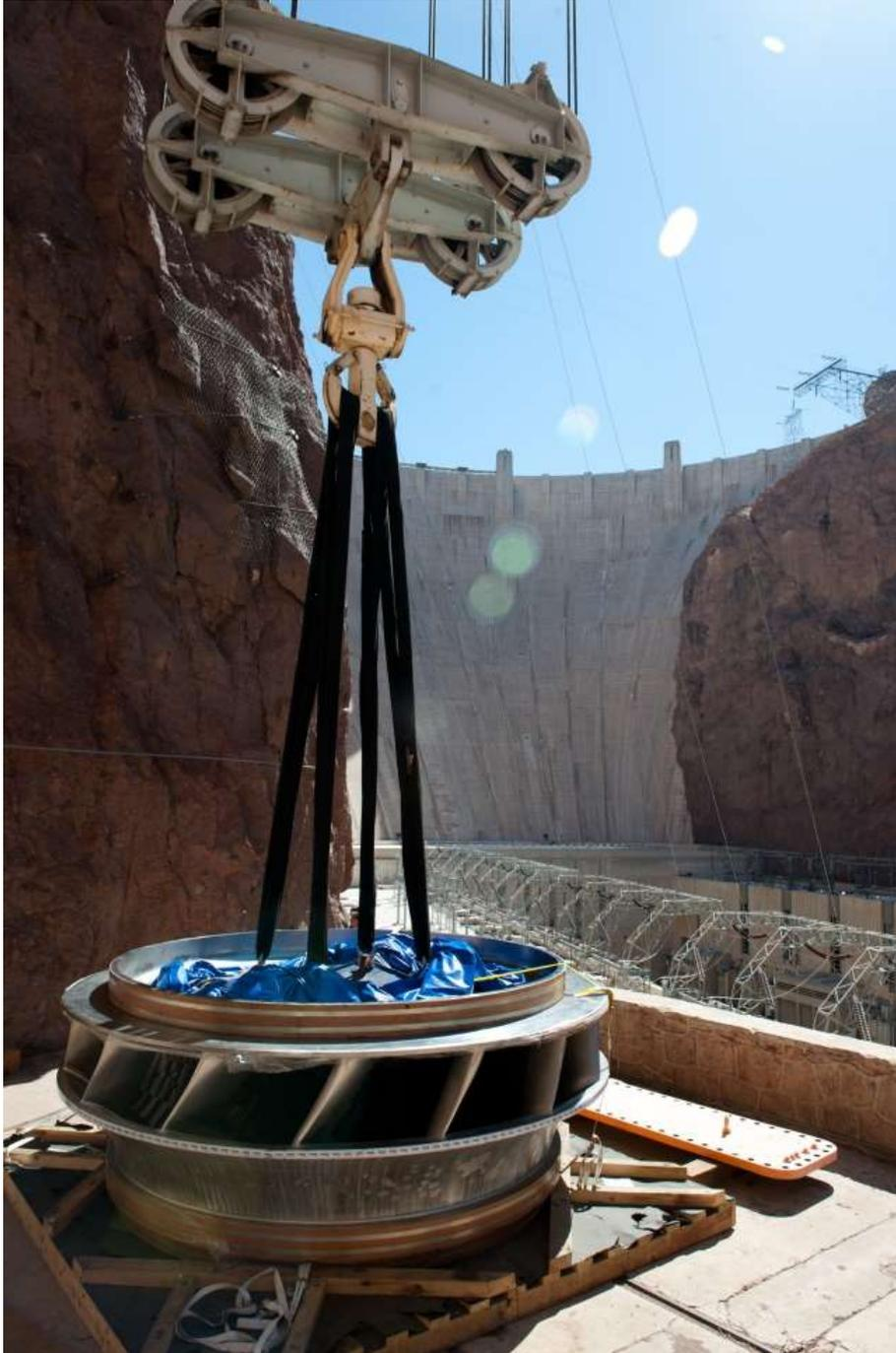
**Figure 3–7. Delivery of a widehead turbine runner for Hoover Dam. The turbine was delivered on a flatbed truck wrapped in a protective tarp. The turbine was flown in using the overhead crane. Date Taken: June 17, 2015.**
