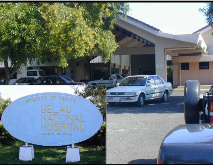
Belau National Hospital
