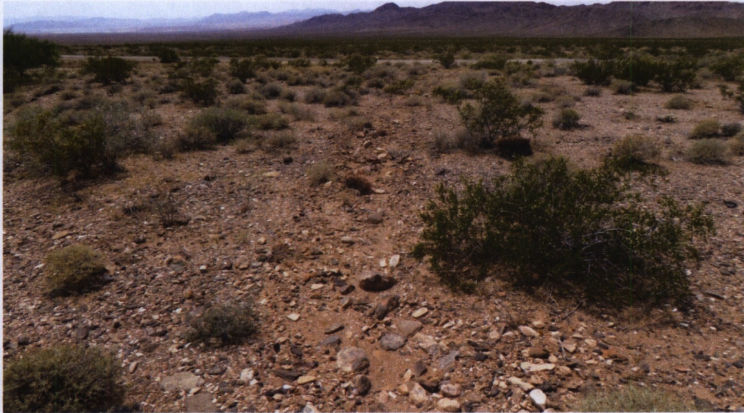
Image 12: Trench #2 and pipe headed toward Gold Butte Road from the tractor and on southwest. Photo looking west. Photographed May 10, 2015.
