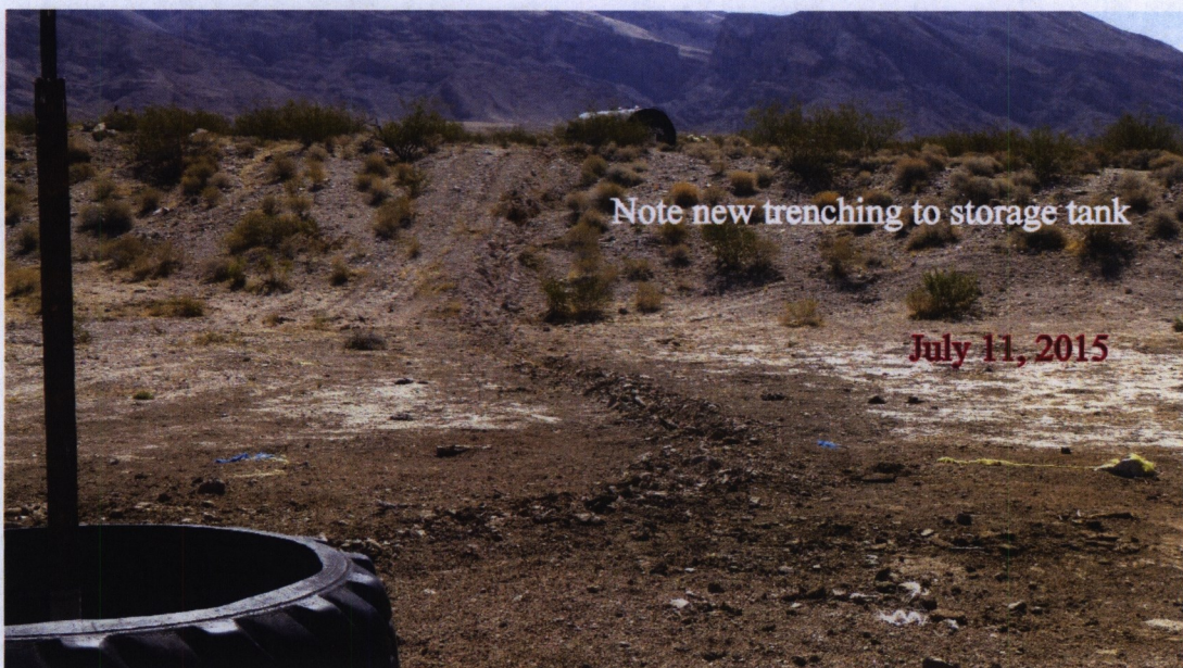
Image 18: Trenching to water tank. Photographed July 11, 2015.
