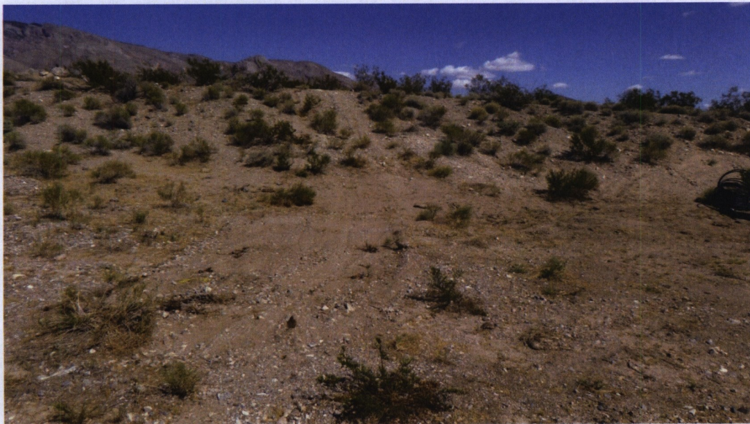
Image 3: Vehicle damage to desert near tank, likely caused in delivering the tank, looking east. Photographed May 10, 2015.
