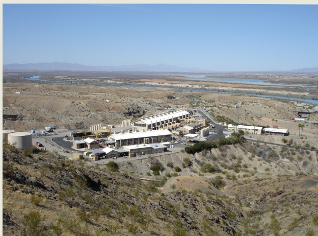
The PG&E Compressor Station sits at the foot of the Chemehuevi Mountains approximately 1,500 feet from the Colorado River.
