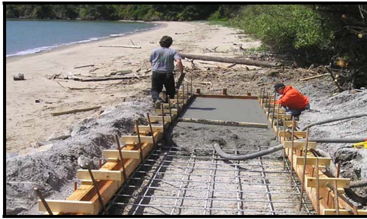
ADA ramp construction at Quarry Beach.
