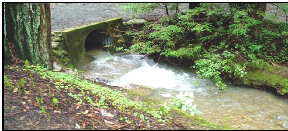
Culvert replacement at McGarvey Gulch to improve Steelhead passage.
