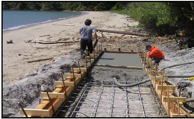
ADA ramp being constructed at Quarry Beach.
