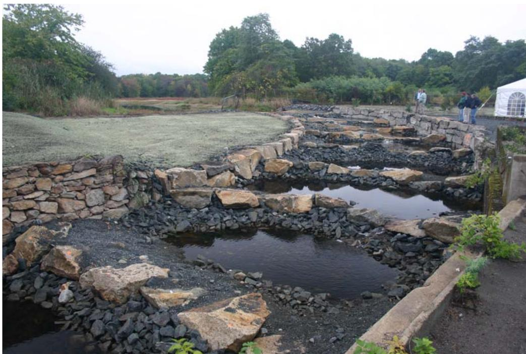
Newly constructed step pool at the former Acushnet Sawmill Dam on the Acushnet River (shown during low flow conditions) will facilitate fish passage and breeding.
