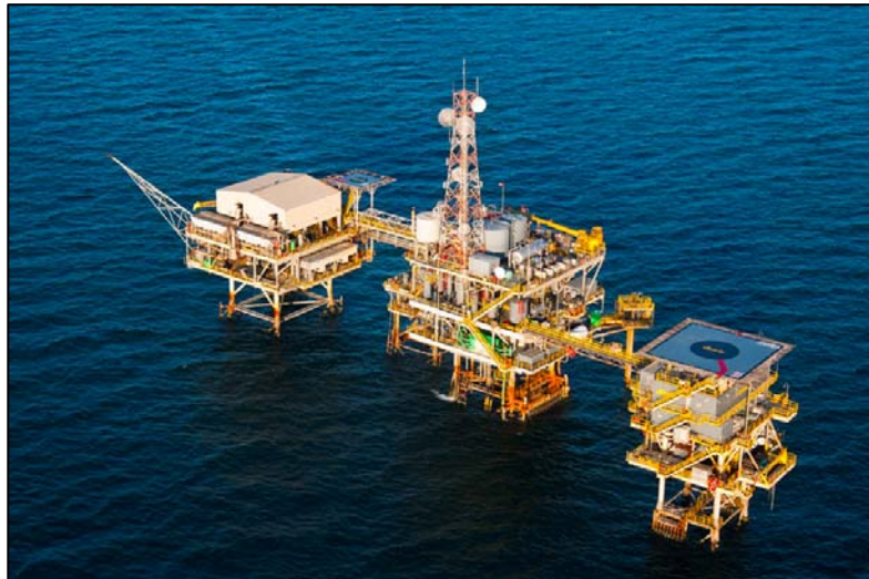
Offshore drilling platform
