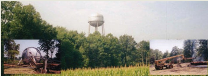
Water Tower 1, once supplying water to the Crab Orchard National Wildlife Area residents, was felled and removed in August 2000.
