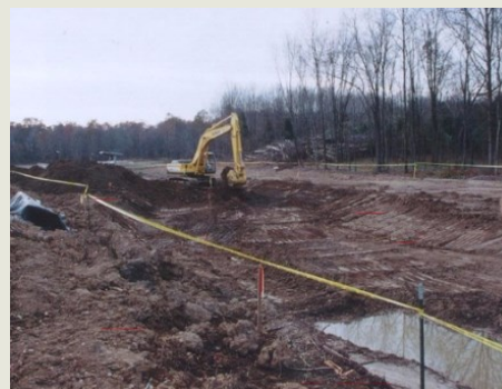
Contaminated soil removal work being completed at Crab Orchard National Wildlife Refuge.
