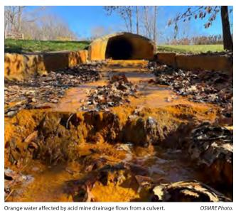
Orange water affected by acid mine drainage flows from a culvert.
