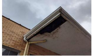
Greyhound Bus Depot, south canopy roof soffit showing deterioration.
