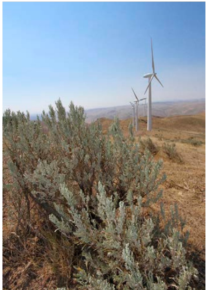
Lime Wind Energy Project in Oregon.
