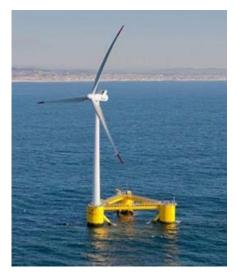
A full-scale prototype of the WindFloat device
