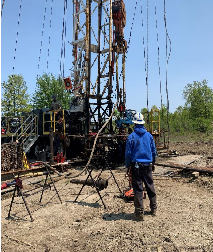
Figure 11: Work underway to plug an orphaned well in Southeast Michigan.
