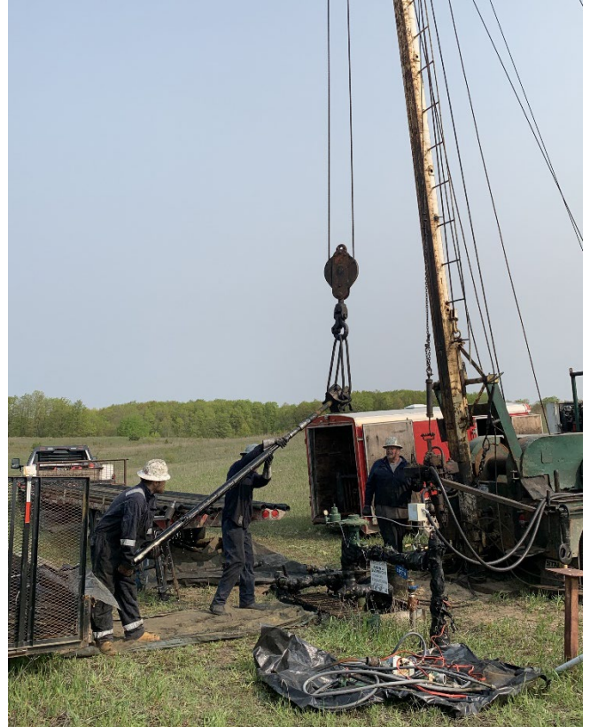
Figure 12: Work underway to plug an orphaned well in Northern Michigan.
