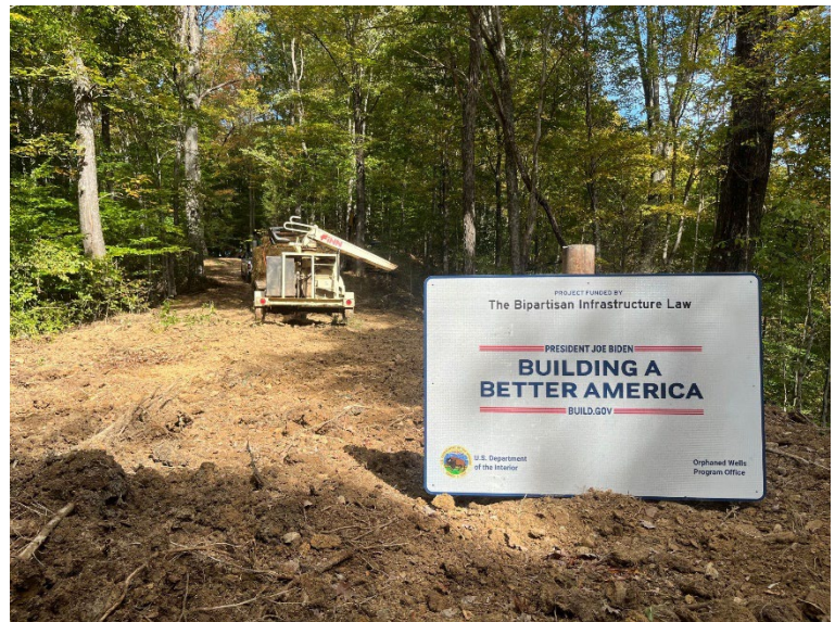
Figure 10: Gauley River National Recreation Area, BIL funded orphaned well site post plugging.
