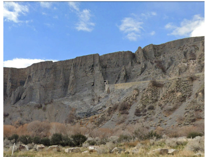
Figure 2: General habitat conditions along the limestone cliffs on the eastern edge of the study area. The spillway and cement roadway can be seen in the middle/right of the photo. Image was taken using Google Earth Street View.
