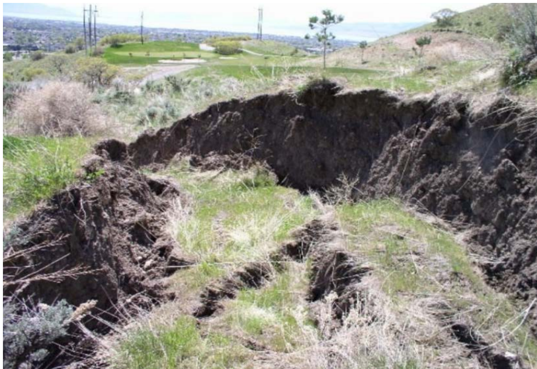
Photo of a Landslide along AA-1 Pipeline
