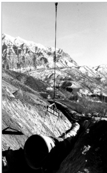
Construction of the Alpine Aqueduct Reach 1
