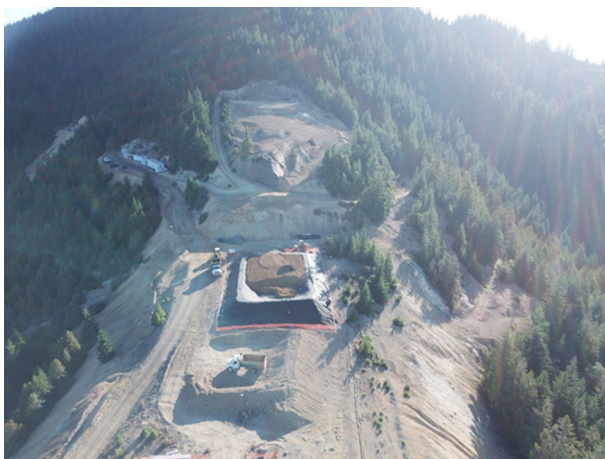
Temporary mine waste repositories being constructed at the site during bulkhead installation. (Photo: John Barber, BLM)
