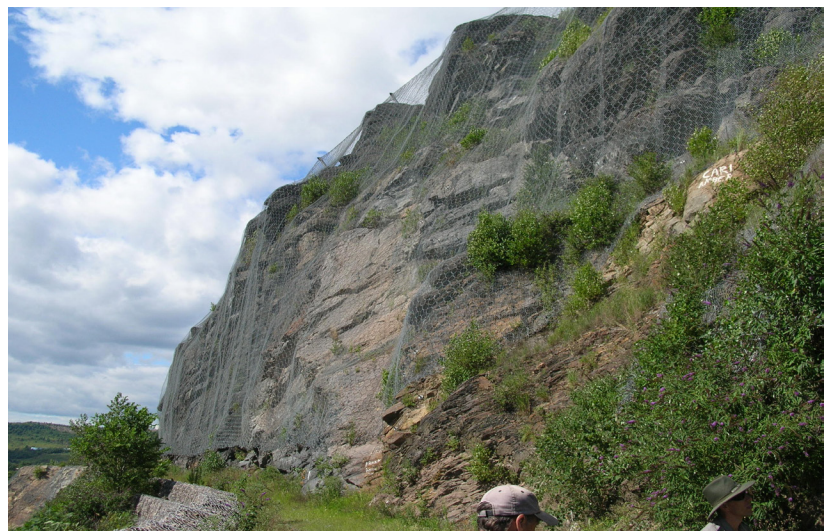
Fencing used to protect hikers from rock slides. (Photo: Greg Nottingham, NPS)
