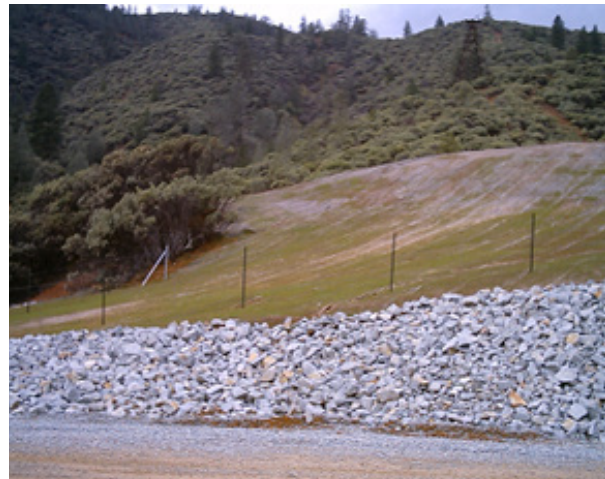
Before and after photos of the excavation, consolidation, and capping of pyrite contaminated soils at the Matheson Ore Transfer Station, near Redding, CA.
