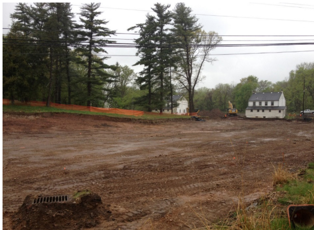
Before: Soil excavation and remediation activity at the Valley Forge NHP. (Photo: NPS)
