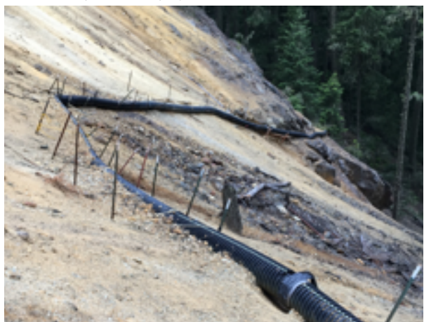
Acid mine drainage diversion system scheduled for replacement in 2019 by BLM to protect watershed water quality. (Photo: John Barber, BLM)
