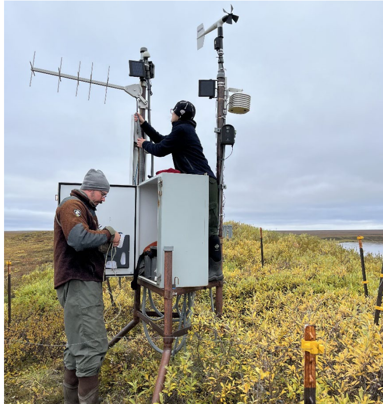
Making final repairs to the Ikpikpuk gage instrumentation
