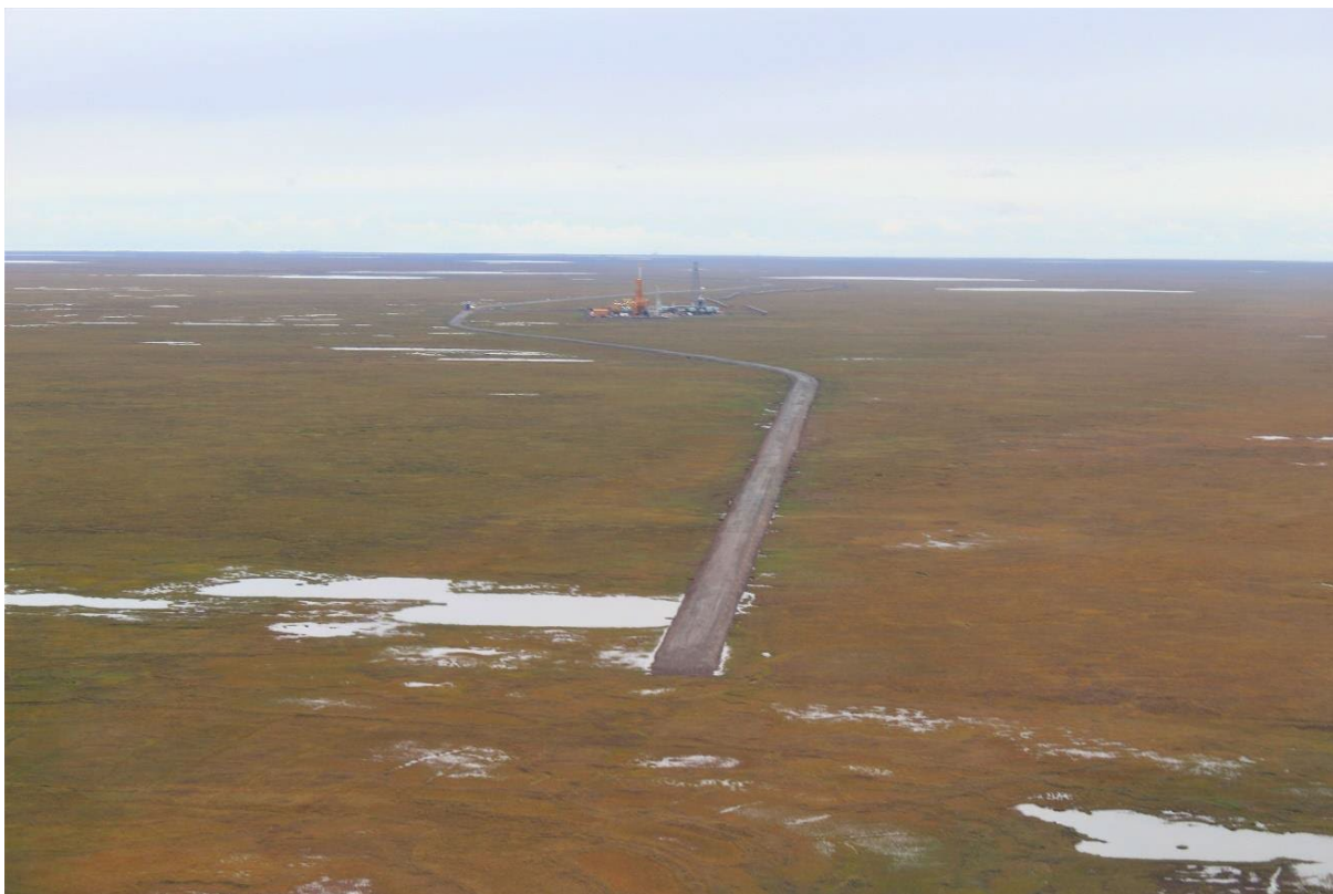
Willow Road Construction, August 2023
