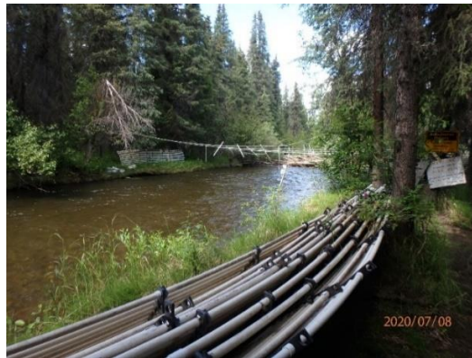
Photo of Tanada Creek weir site
