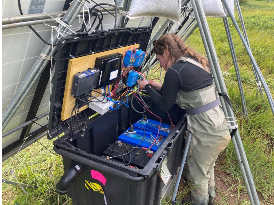
Figure 3. SCA intern Chaney Haavik installs electronics at the Sitkoh Lake weir.
