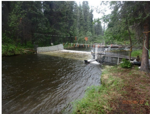
Tanada Creek Salmon Weir, 2023
