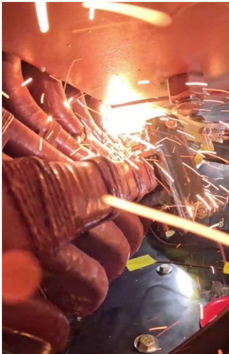
IMAGE SHOWING A SIDE VIEW OF THE FAULT CREATED FOR THE EXPERIMENT PRIOR TO DEPLOYMENT OF THE FIRE SUPPRESSION SYSTEM. PHOTO: BOR
