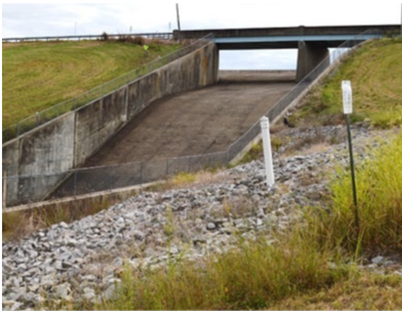
Little Grassy Dam Service Spillway, Crab Orchard, NWR, IL. Planning for rehabilitation is currently underway with a cooperative agreement between Region 3, NWRS and the USACE. Credit: USFWS
