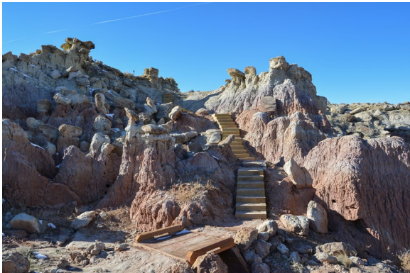
Completed construction work on Gooseberry trail.
