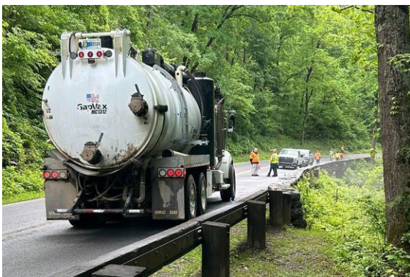
Construction work on Newfound Gap Road. Photo Credit: NPS
