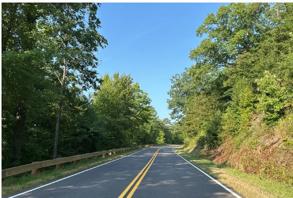
Completed Foothills Parkway in Great Smoky Mountains National Park. Photo Credit: FHWA
