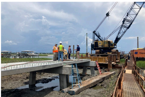
Repairs to the dock at Fort Moultrie in progress.
