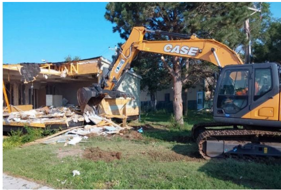
Demolition activity at a BIE-funded educational facility. Photo Credit: EQMS
