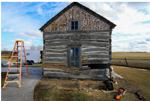
MAT member restoring the historic Palmer-Epard Cabin. Photo Credit: NPS/Robert Hartwig
