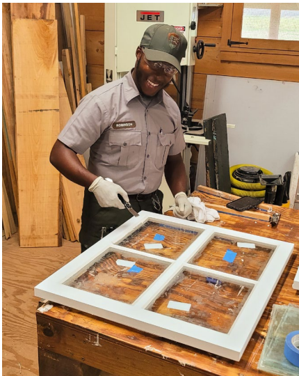
A member of a Maintenance Action Team glazing a window.
