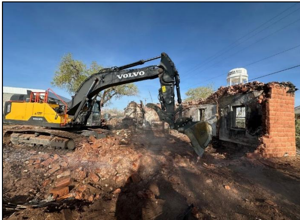
Figure 4 – Demolition in progress at Tuba City Boarding School. Photo Credit: EQM
