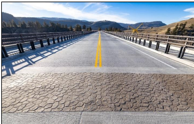
Figure 3 – Completed Yellowstone River Bridge. Photo Credit: NPS
