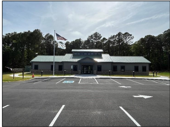
Figure 6 – Completed visitor contact station at Prime Hook National Wildlife Refuge. Photo Credit: USFWS
