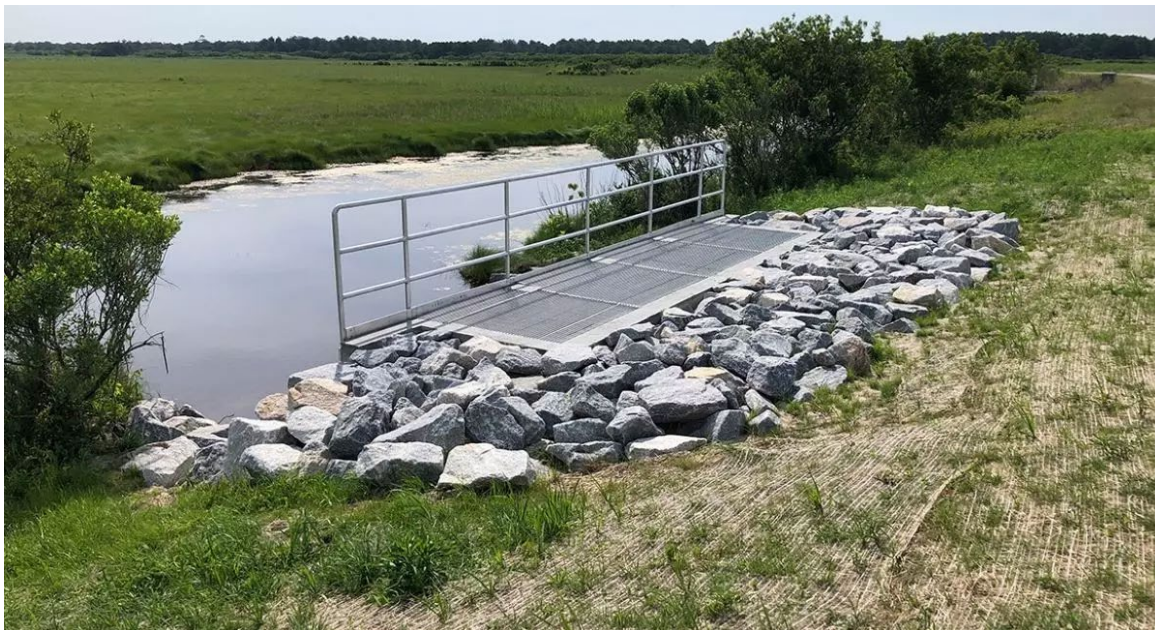
Wetland managers use water control structures like this one to help regulate water levels to control exotic invasive vegetation at Cedar Point and Ottawa National Wildlife Refuges in Ohio. Photo: USFWS.
