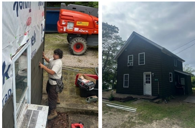
GAOA Funded Maintenance Professional Replacing Siding on a Quarters building at Ninigret NWR. Image: USFWS
