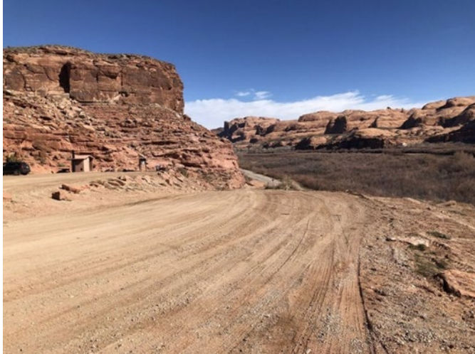
Moab Recreation site road after reshaping.
