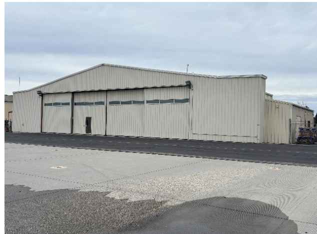
Building 405 Hanger at the National Interagency Fire Center
