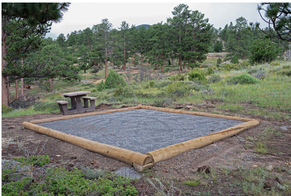
New tent pad at a campsite in Rocky Mountain National Park. Photo Credit: NPS
