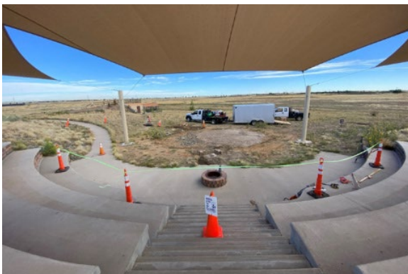
Visitor Center Stage replacement in progress. Photo Credit: USFWS
