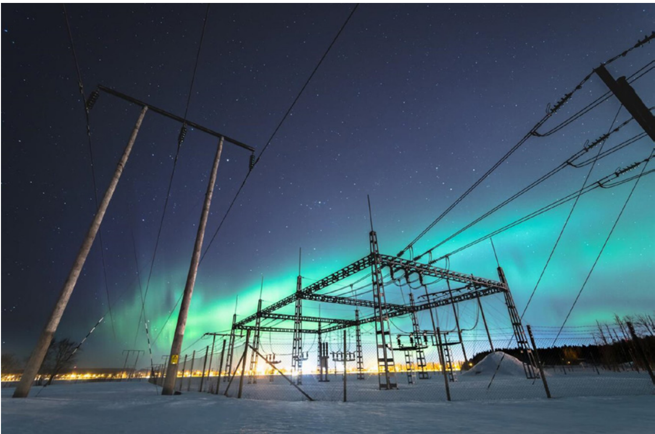
To better understand ground-level magnetic-storm hazards, USGS scientists developed a new map of geoelectric fields. In some areas, expected field strengths would be enough to stress or damage high-voltage transformers and potentially lead to massive power outages.
