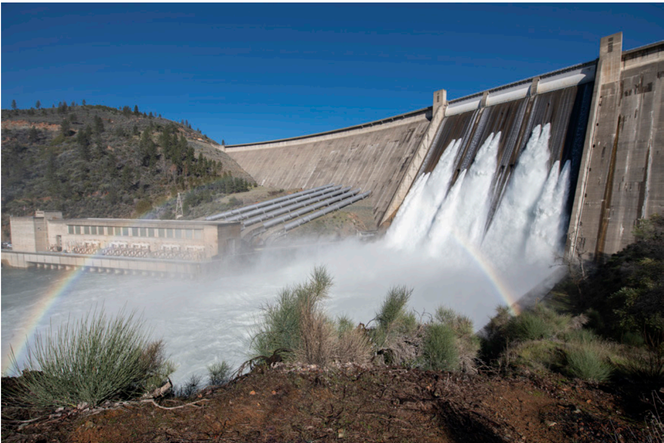
Shasta Dam in flood operations with 10 river valves open, letting water flow into the Sacramento River.
