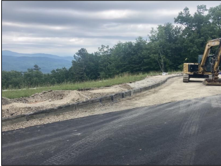
Figure 10 – Workers resetting the stone curb along a pullout on Foothills Parkway in Great Smoky Mountains National Park. Photo Credit: NPS
