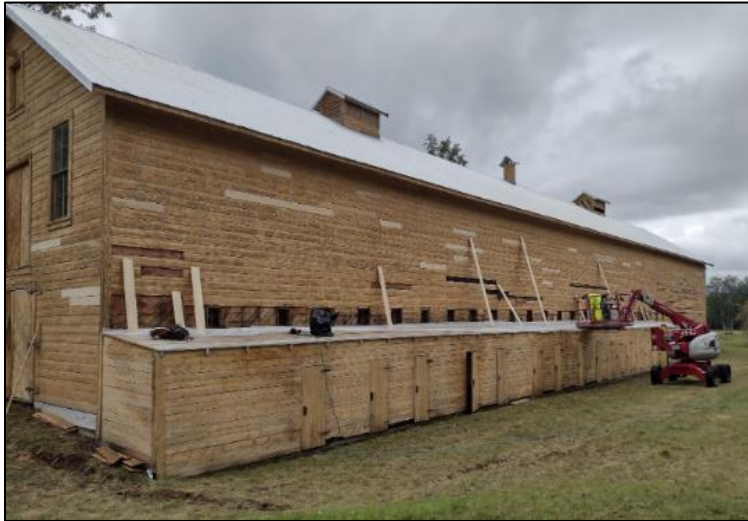
Figure 5 –Construction worker replaces rotten boards with new siding on the Mule Barn at Fort Egbert National Historic Landmark. Photo Credit: BLM/Stuart Mitchell
