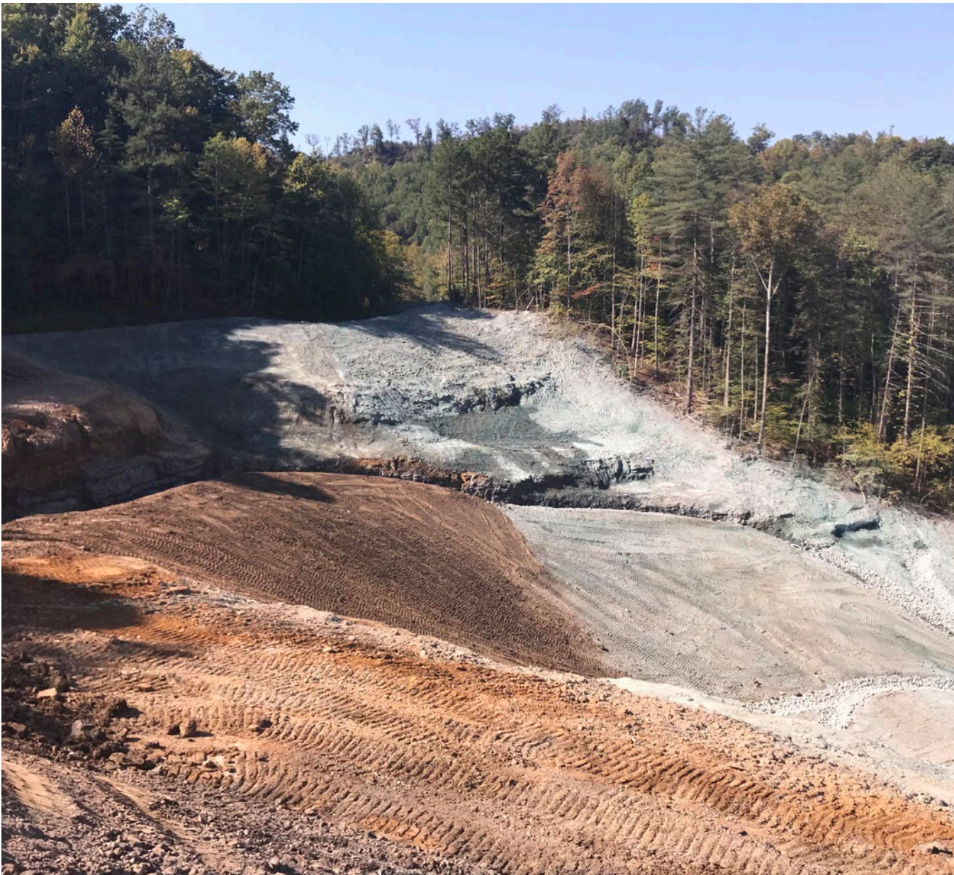
A seeded and graded hillside at a reclaimed abandoned mine land site in eastern Kentucky.
