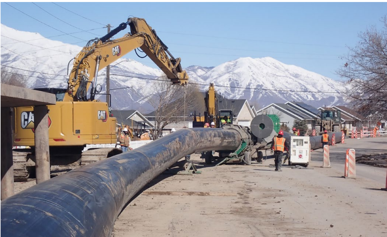
Spanish Fork-Santaquin Pipeline fusion of 42-inch high-density polyethylene sections.
