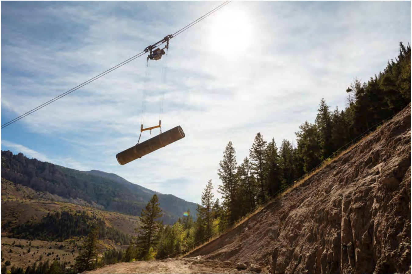
A cableway crane is used to hoist a 40-foot-long section of 84-inch-diameter welded steel pipe from the valley floor for installation on the steep canyon slope as part of the North Fork Siphon Replacement Project, Central Utah Project.
