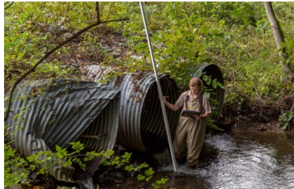
Photo: Assessing aquatic organism passage at a road-stream crossing in Maryland. Photo credit: Steve Droter/USFWS
