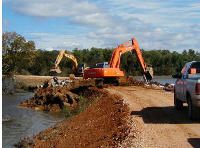
Figure 3. Typical Picture of Levee Rehabilitation
