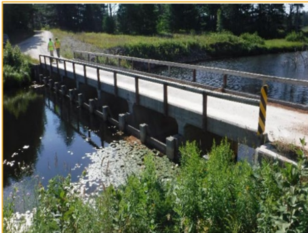
Figure 1. Seney NWR Auto Tour Bridge
