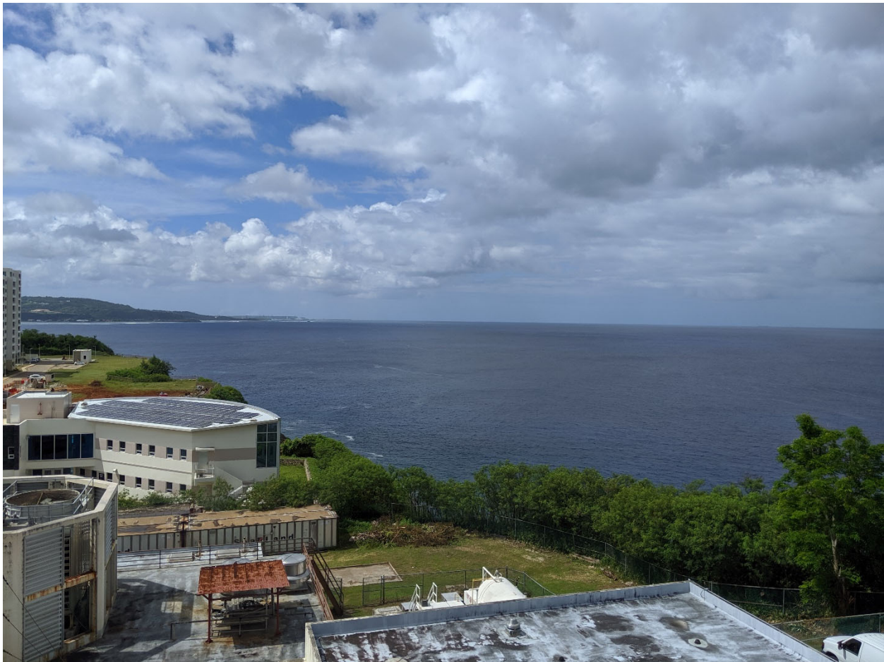
View from roof of B-wing overlooking the central plant and showing the proximity to the Pacific Ocean
