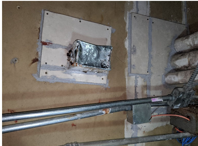
View through access panel/grille inside patient bedroom soffit/plenum space
