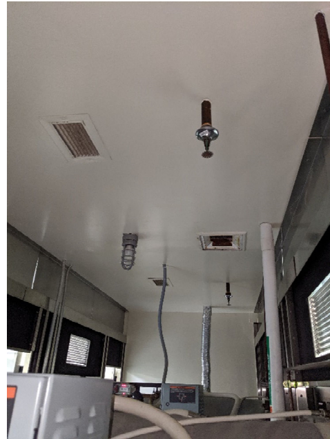
Inadequate exhaust in sterilizer equipment room
