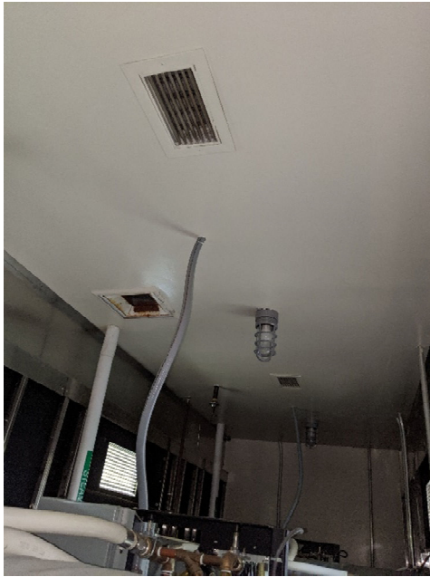
Inadequate exhaust in sterilizer equipment room
