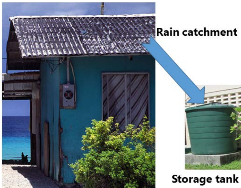
Figure 2: Private rainwater catchment and storage system (house photo is courtesy of Stefan Lins, used under creative commons, and tank photo is from Reclamation 2020).
