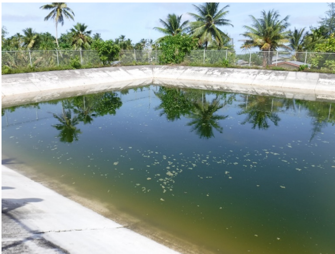
Figure 10: Raw water temporary holding pond at WTP A (Reclamation, 2020).
