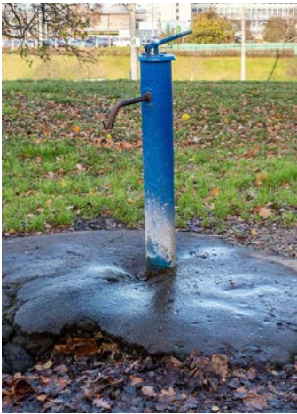
Figure 41: Public standpipes (photo used is courtesy of Uladzimir under a Creative commons license).
