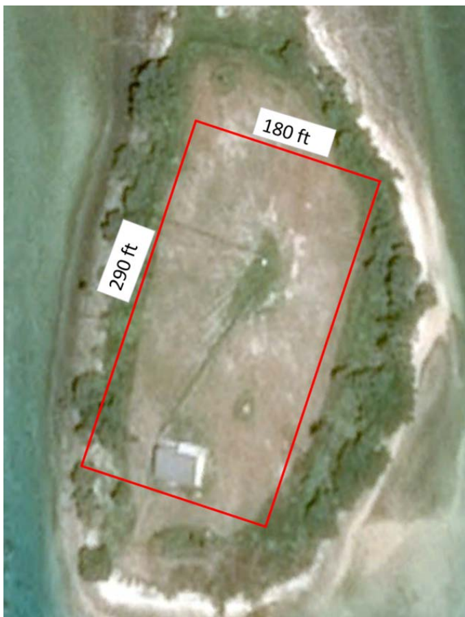
Figure 43: Bokiur Island ground reservoir site.
