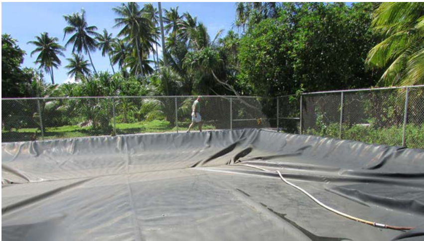
Figure 4: Laura Reservoir for untreated water prior to treatment at Laura WTP (Reclamation photo 2020).
