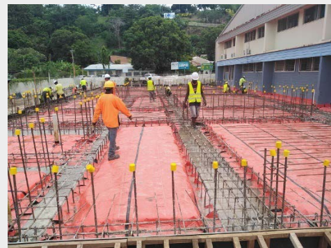
Full under-slab termite protection layer in high-risk area
