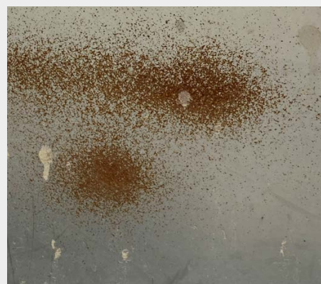
Corrosion on stainless steel caused by contamination with carbon steel particles.
