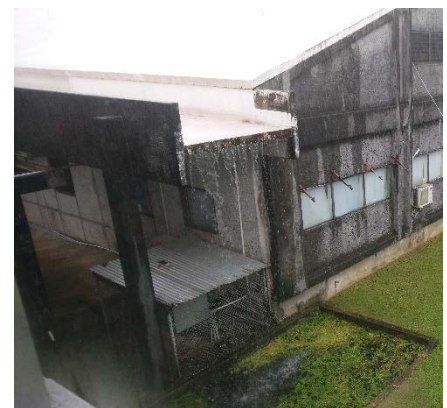
Figure 4-1: Wide gutter located in Pohnpei. Photo supplied by USACE
