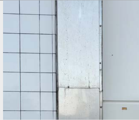
30-year-old 316 stainless steel faring well in tropical conditions
