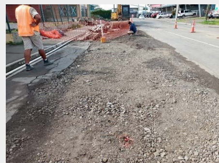
Road repairs and trench reinstatement
