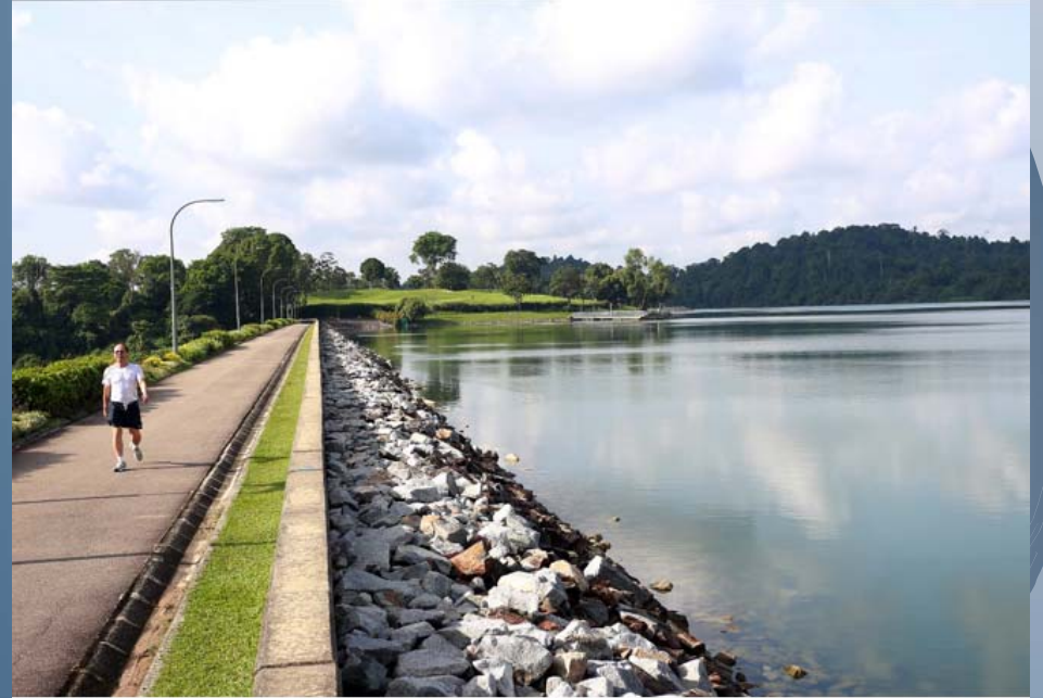
LOCAL CATCHMENT, UPPER PEIRCE RESERVOIR - SINGAPORE
